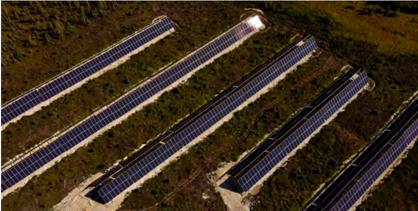
An aerial view of Sree Vyah showing the mono-crystalline panels positioned east and west to maximize solar generation during the Arctic summer. Photo by Caleb Charlie
