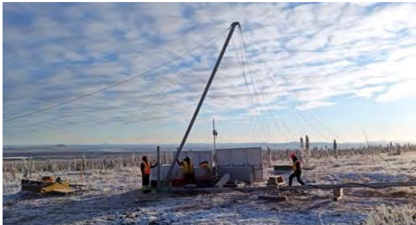
Erecting the Meteorological Evaluation Tower (MET) on Mountain Road.
